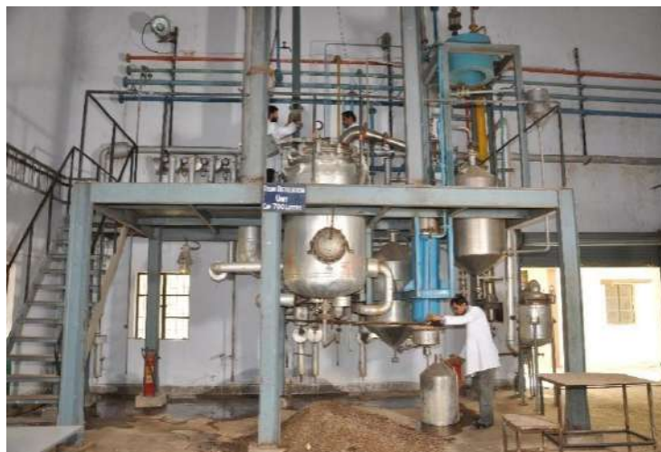
Steam Distillation Unit at Pilot Plant
